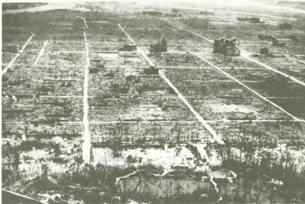
Figure 1.1 Panoramic view of Hiroshima following the atomic bomb explosion of August 6, 1945. In the few standing structures of reinforced concrete, the interiors were totally gutted and burned. Reproduced by permission of Popperfoto
