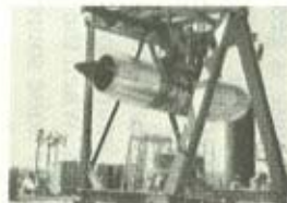
20-LOBE EJECTOR SUPPRESSOR FOR 727 AIRPLANE
